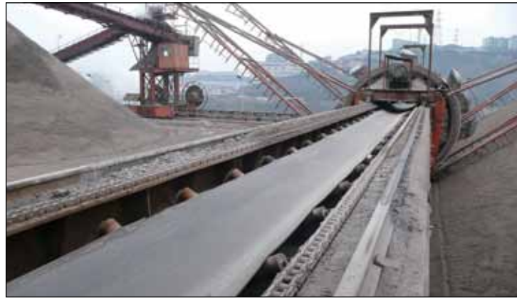
Bulk material conveyor chains
