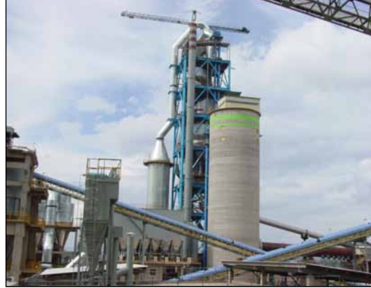
Conveyor chain for cement mill
