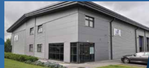
Donghua Limited - United Kingdom UK distribution centre
